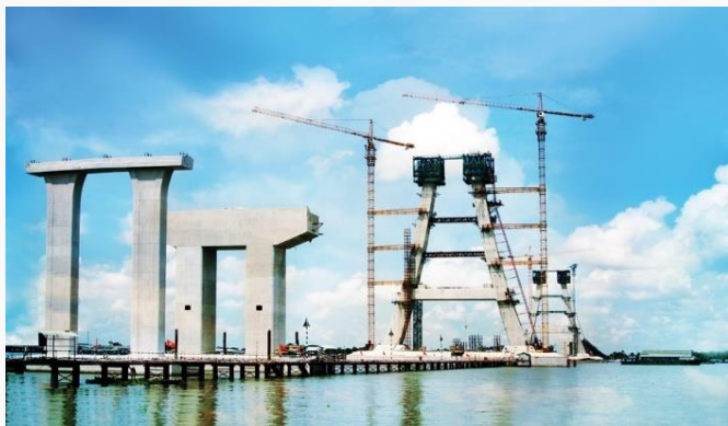
Vam Cong bridge project China road and bridge corporation
