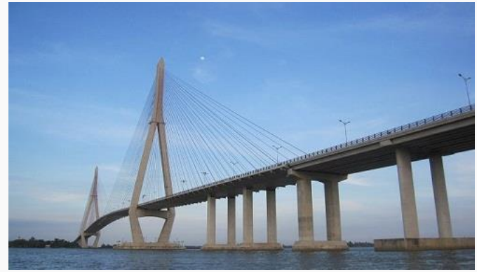
The Ninth bridge in Can tho province China State Construction (SEA) Corporation
